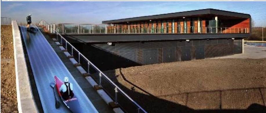
The design development process involved hydraulic modelling and full scale testing to optimise the design and minimise the energy requirements
